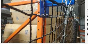
The flue space between racking systems is often an area that sees a high volume of product falls and damages that workers are unable to access. Our Rack Netting System can be installed within this space to help reduce product loss and keep products from getting mixed up with another pallet load.
